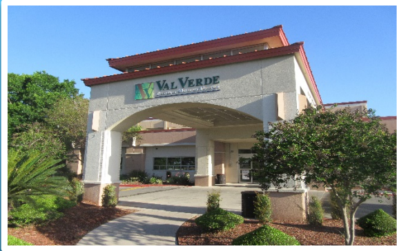
Val Verde Regional Medical Center Del Rio, TX
