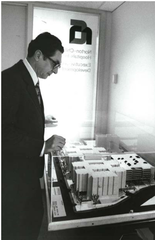
Viewing a model of the new building, 1970
