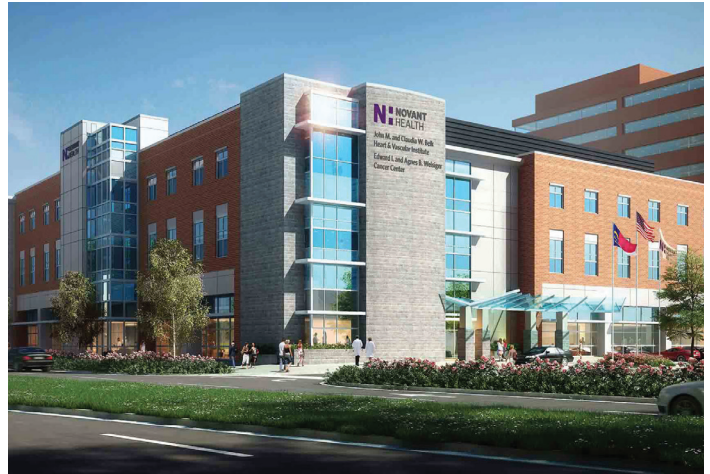
Novant Health Presbyterian Hospital in Charlotte, N.C.
