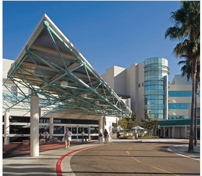
Sharp Grossmont Hospital – La Mesa, CA
