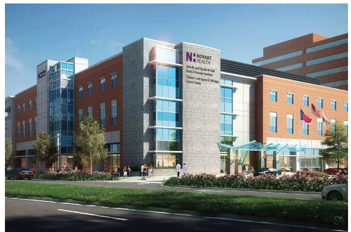
Novant Health Presbyterian Hospital in Charlotte, N.C.
